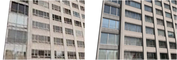
Figure 9. Left: input image of low quality. Right: enhanced results exploiting semantic understanding of the façade structure.
